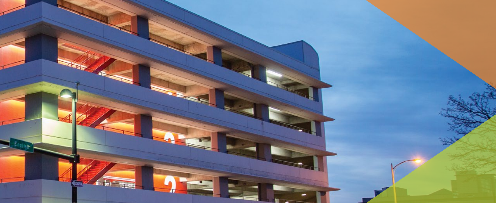
The Broadway Autopark Apartments
